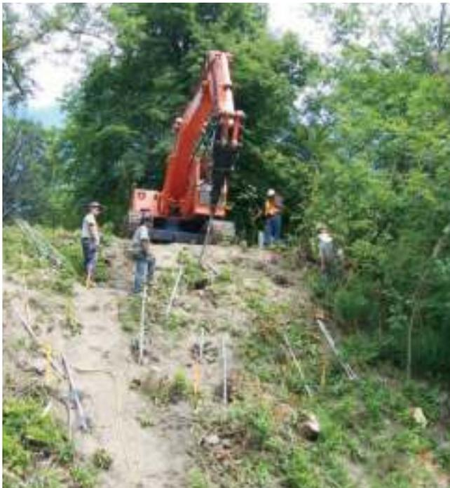
in the installation, Soil Screw anchors provide required capacity immediately upon installation.
