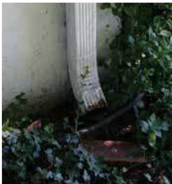
Poor drainage is a major factor contributing to expansive soils due to over saturation.
