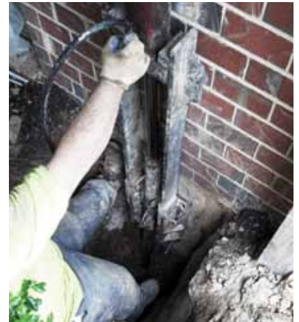
UNDERPINNING INSTALLATION
