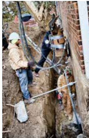
UNDERPINNING INSTALLATION
